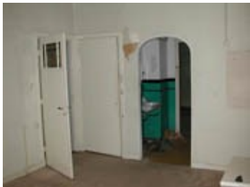
Photo of the old entrance from bedroom 2.
